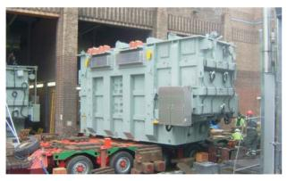
Although the Bankside Power Station ceased operation several decades ago, the substation continued to operate and remains an important part of London's electricity network. The  $\pm 60$  million refurbishment of the substation included many substation upgrades, 6 power transformers from Wilson Transformer Company in Australia and an engineered heat reclamation system that used the losses of the transformers to supplement the heating and hot water requirements of the adjacent Tate Modern.
